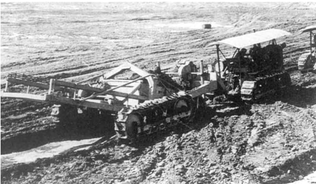
Two views of the telescopic scraper at Philbrook Dam. The one in the top photo appears to be dumping its load of dirt while the one in the bottom photo is scraping up a load as is evident from the smooth trench behind it. The Bancroft Library, University of California, Berkeley.
