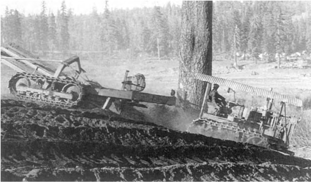
Two views of the telescopic scraper at Philbrook Dam. The one in the top photo appears to be dumping its load of dirt while the one in the bottom photo is scraping up a load as is evident from the smooth trench behind it. The Bancroft Library, University of California, Berkeley.
